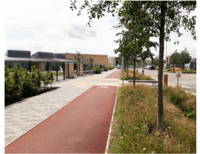
Example of dedicated space provided to cyclists and pedestrians separated from the carriageway with tree planting and sustainable urban drainage.
