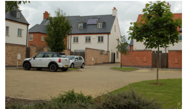
Courtyard parking with planting and overlooking
