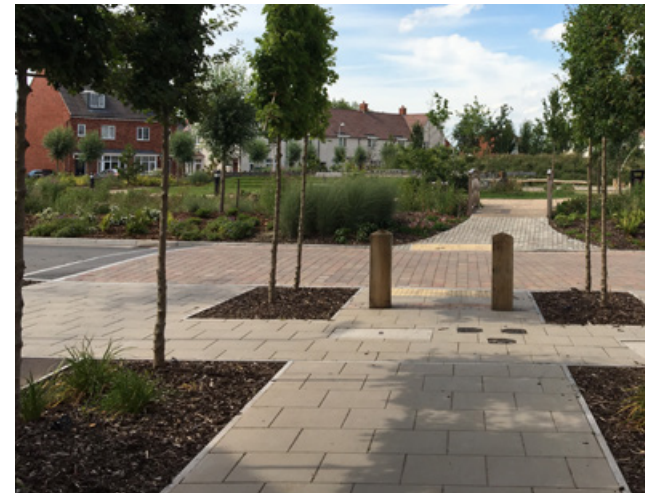
Example of a junction between a street and a footpath where a raised table and textured paving gives priority to pedestrians
