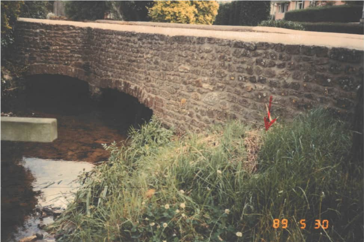
Fore Street Bridge (Downstream Face)
