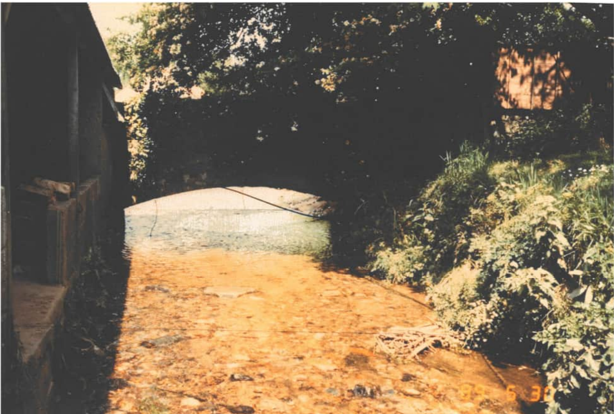
Bridge House, looking upstream, flood boards in photo were ineffective as water gained entry at side and front of the property
