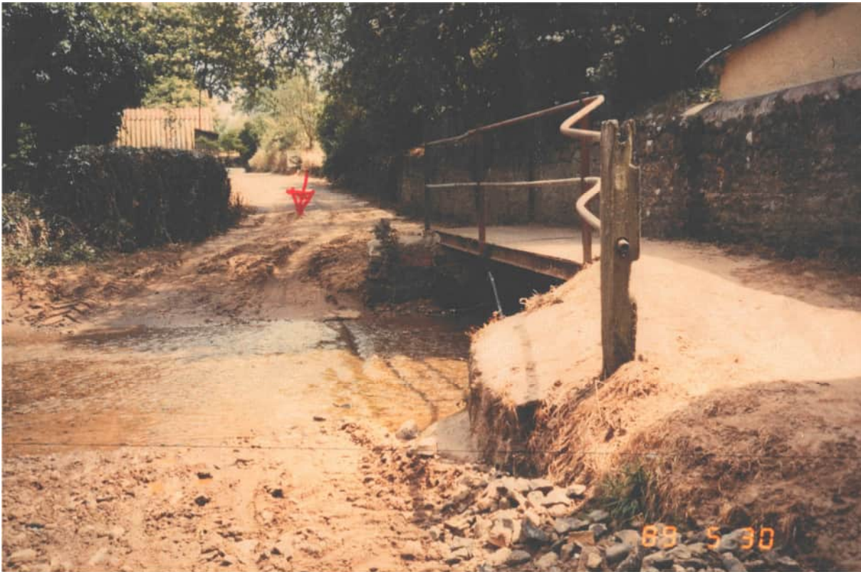
Bridge Adjacent to Brook House
