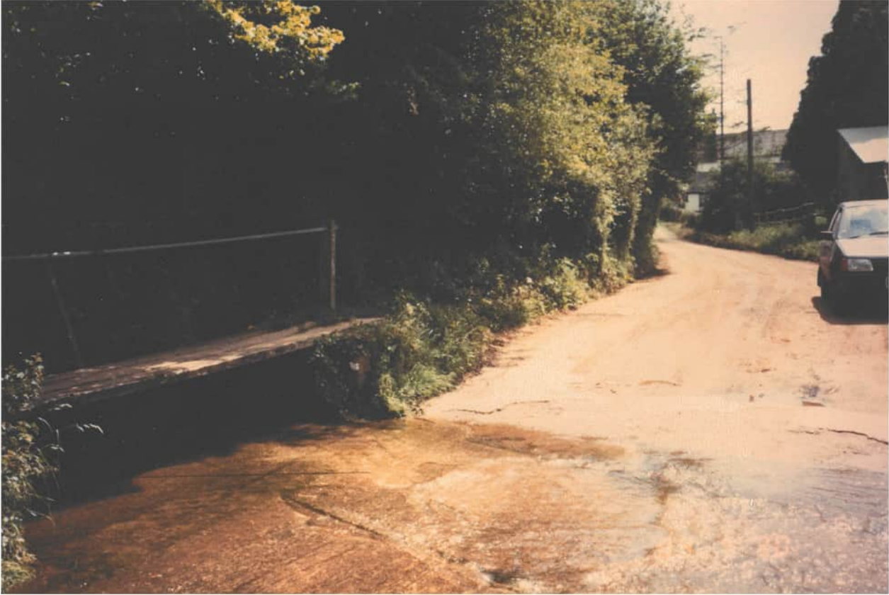
Goodiford Farm – Flood water overtopped the footbridge
